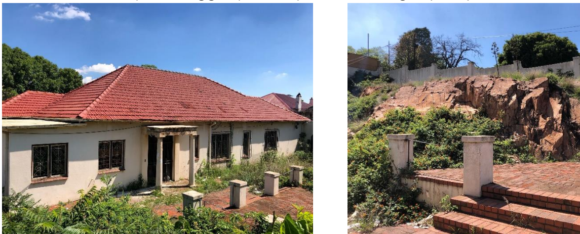
South facade, and exposed koppie on the southern boundary: photo by Brett McDougall (2019)
