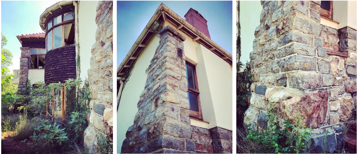
Details of the north facade, including the impressive stone quoining and buttresses: photos by Brett McDougall (2019)
